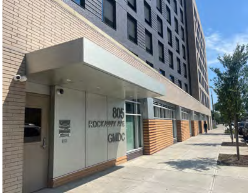
GMDC Brownsville Industrial Center at Bridge Rockaway in Brownsville, Brooklyn
